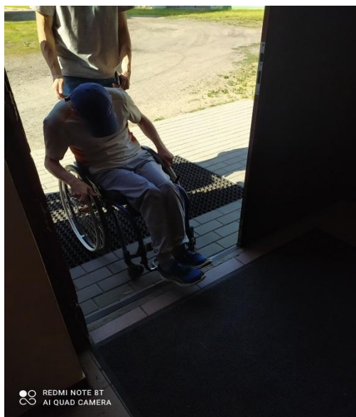
The threshold at the entrance to the hall building Small toilet rooms do not allow wheelchair access
